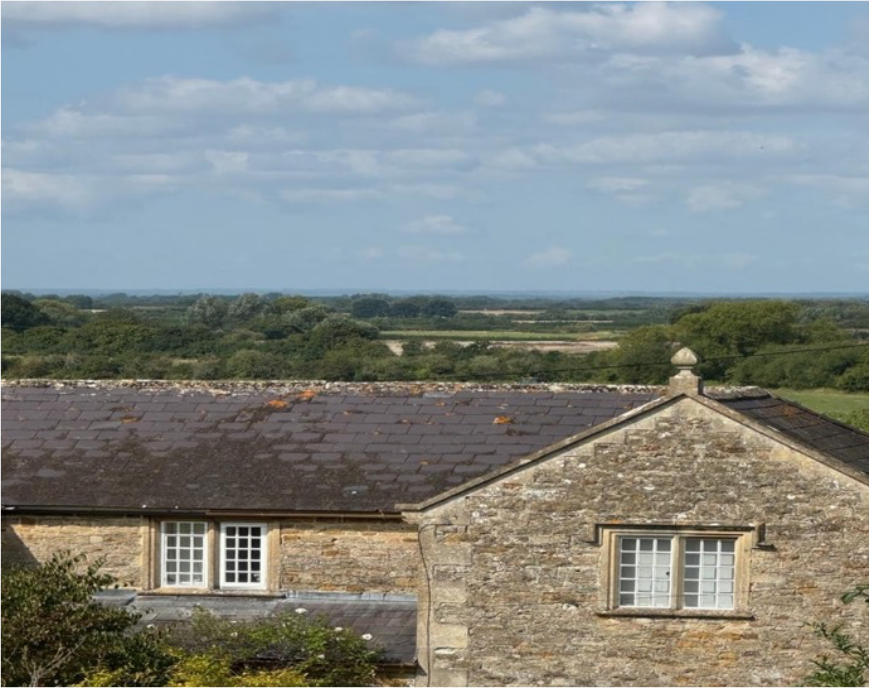
Site excavation from National Trust building, Estate Yard, Coleshill.
